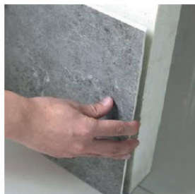
6. Install the cut SPC panels at the edge
