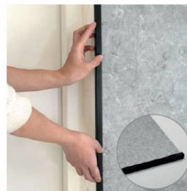
7. Use the end cap to finish the edge
