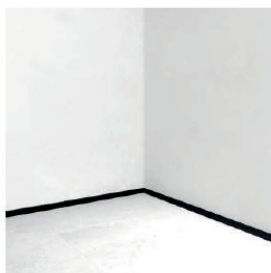
1. Ensure the installed wall is smooth and clean
