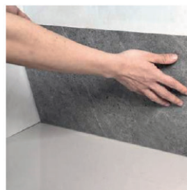
3. Install SPC wall panels
