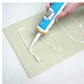
2. Gluing SPC wall panels
